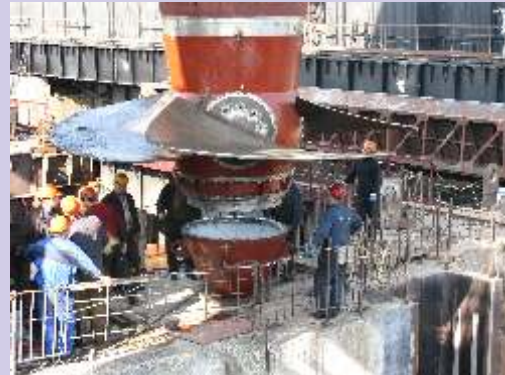
Kamskaya HPP (Russia): Hydro Turbine under Plant Unit No. 17 with Output of 26 MW, with Ecologically-Clean Runner – Hydro Turbine Rotor Mounting. (2011)
