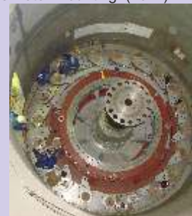
Kamskaya HPP (Russia): Hydro Turbine under Plant Unit No. 17 with Output of 26 MW, with Ecologically-Clean Runner – Hydro Turbine Rotor Mounting. (2011)
