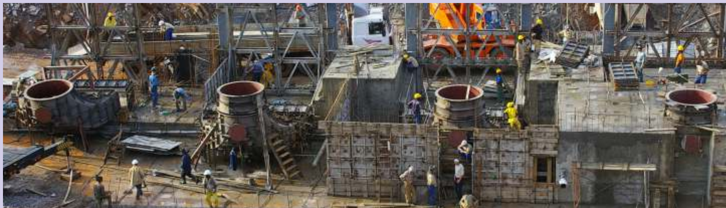
Chicapa HPP (Angola): Mounting of Draft Tubes at Site. (2006)
